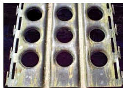
A section of a P.S.P. (Pierced Steel Plank), also known as Marston mat.
