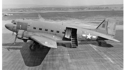
Temporary runway constructed with P.S.P.
